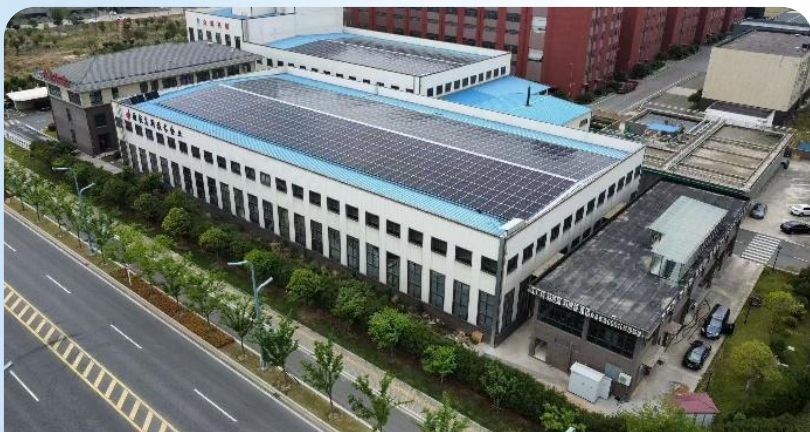
7.4 MW Yangzhou Huiteng Power Distributed PV Project
